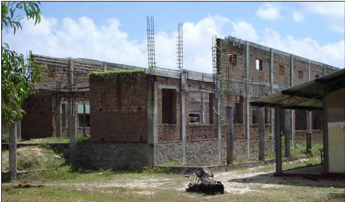
Arts Theater on construction
