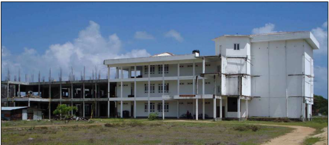
Science Complex on construction
